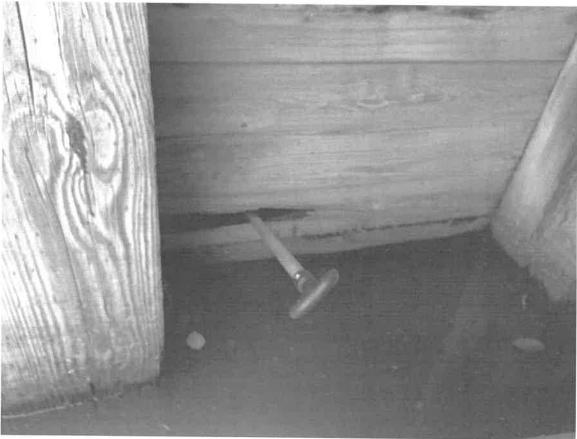
IMG_2110 The oar went over 3' into the cavity at the west end bent.
