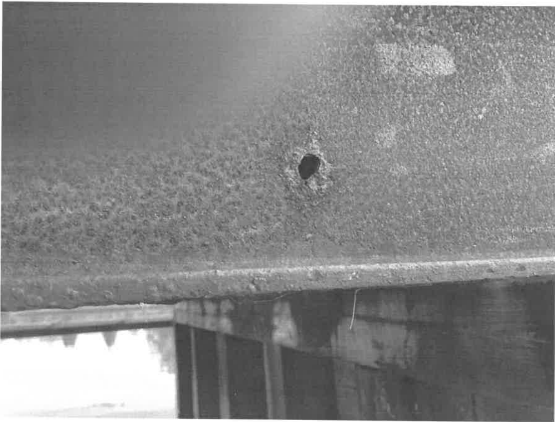
The hole is now completely open through the web.
