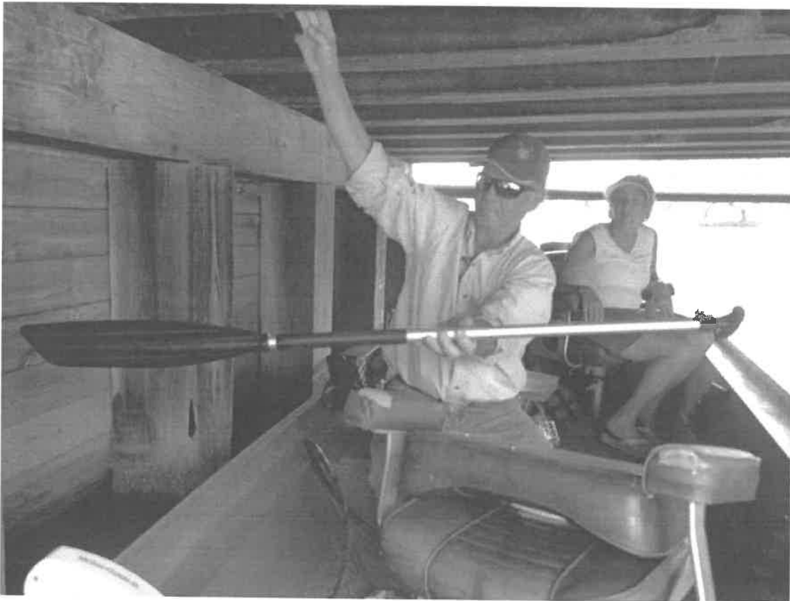
IMG_2110 The oar went over 3' into the cavity at the west end bent.
